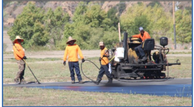
Now, every time you taxi out or in, you'll know how they got those markings down in the "kill zone."
