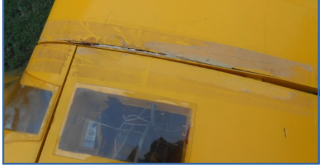
Photo 4: Removing the top sheeting revealed a pretty sparse structure with no reinforcing. Little wonder that end rib worked itself loose.
