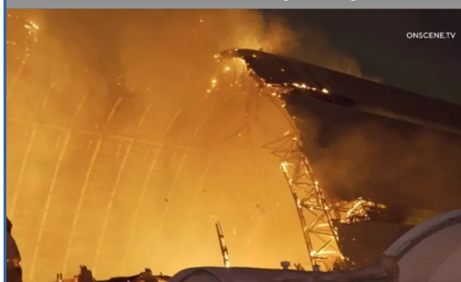
By Wednesday morning the fire was finally under control but the hangar was a total loss.
