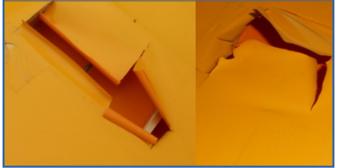
Photo 9: Left horizontal stab will need to be reattached & vertical & horizontal stab braces installed.
